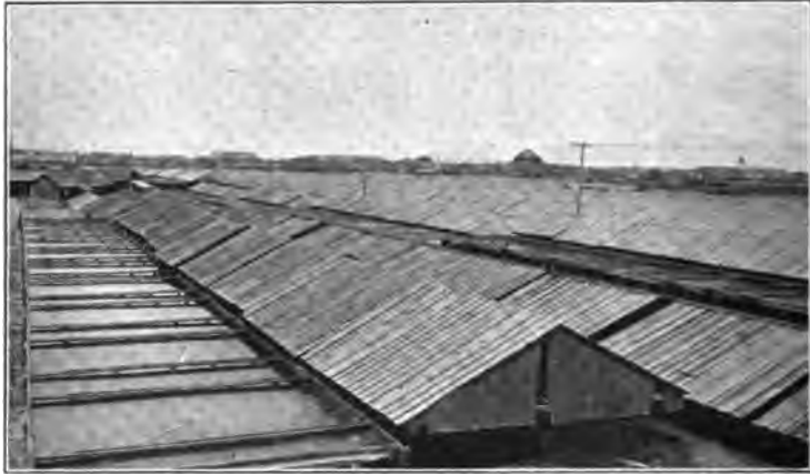
FIG. 1191. — Syracuse salt works. The salt is obtained from the Salina brines, and separated both by solar and artificial evaporation.
